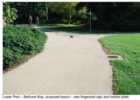
Lower Park – Bethune Way, proposed layout – new fingerpost sign and marker plate.
